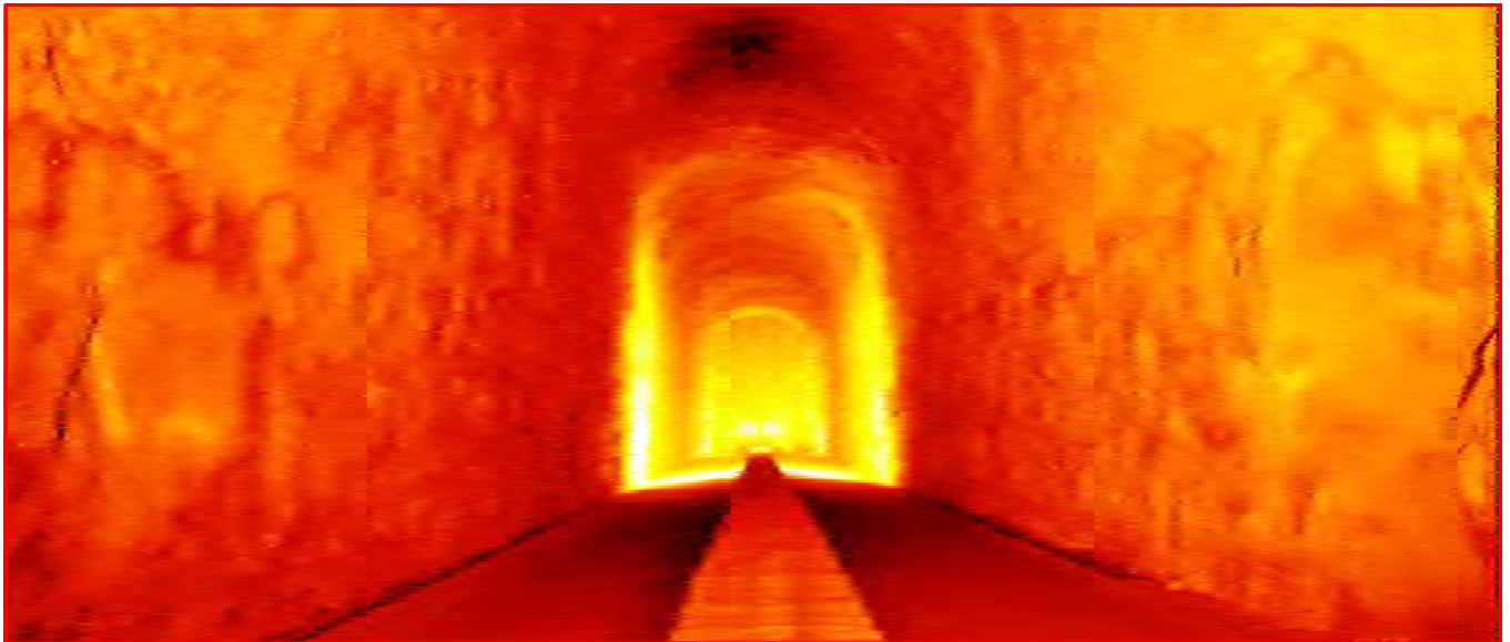
View of the Access Tunnel facilities at Visakhapatnam
