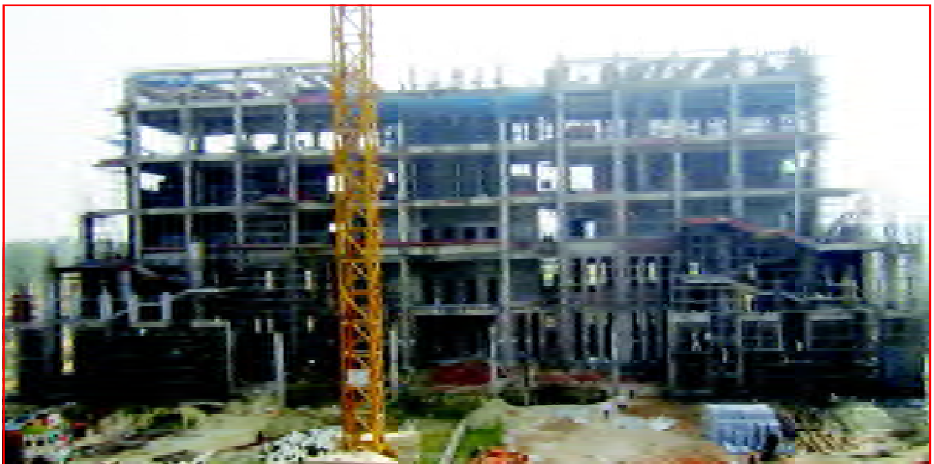
RGIPT, Rae Bareli Campus under construction
