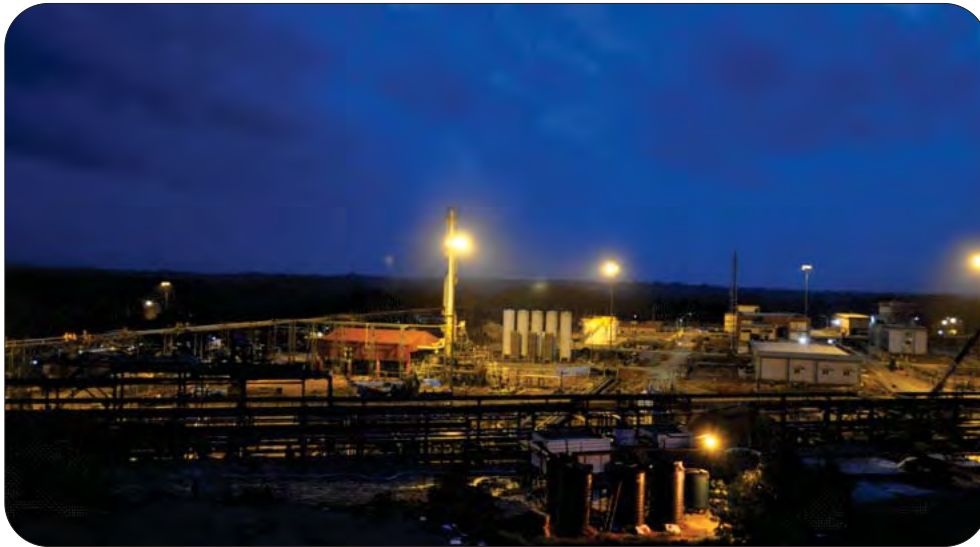
View of the aboveground facilities at Padur
