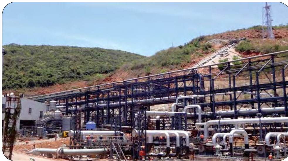
View of the aboveground facilities at Visakhapatnam
