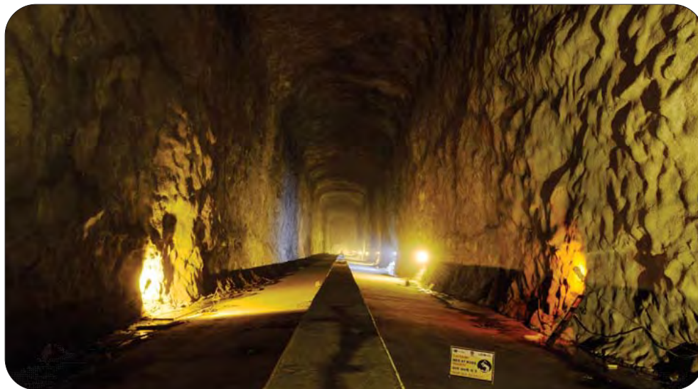
View of one of the four cavern galleries at Mangalore
