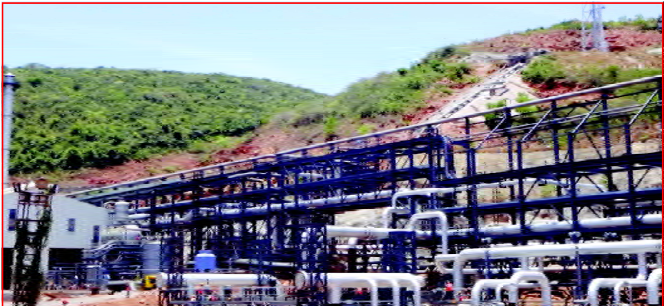
View of the aboveground facilities at Visakhapatnam
